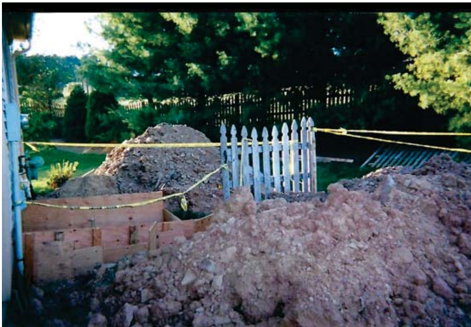
Basement being built, digging for outside Bilko Door
