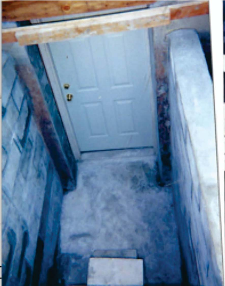
Bilko Door construction
